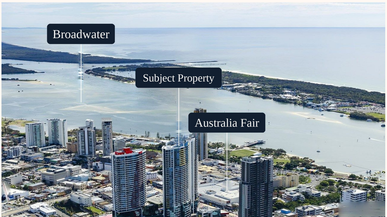
Tower 2 beside Australia Fair, looking north across the Broadwater. Locations indicative.
